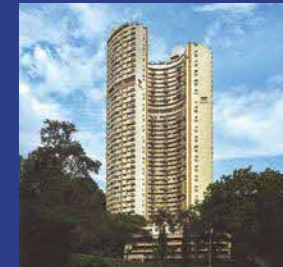
Pearl Bank Apartments, 2014 Courtesy of Archurban Architects Planners Pte Ltd
