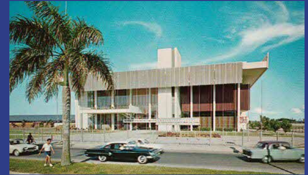
Singapore Conference Hall and Trade Union House, c. 1970 Collection of the National Museum of Singapore, National Heritage Board, 2008-04101
